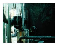
Here, a dock door was left open overnight. The extreme temperature caused freezing of the overhead water supply to the hydrant. This resulted in considerable leakage from the pipe.
