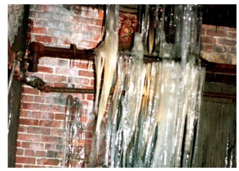
The plan to increase minimum heat in this idle building was far from adequate and resulted in extensive freeze damage.
